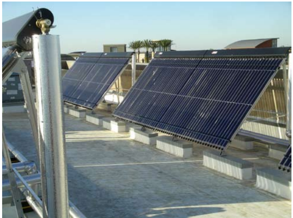
Figure 4 Evacuated tube collector array
