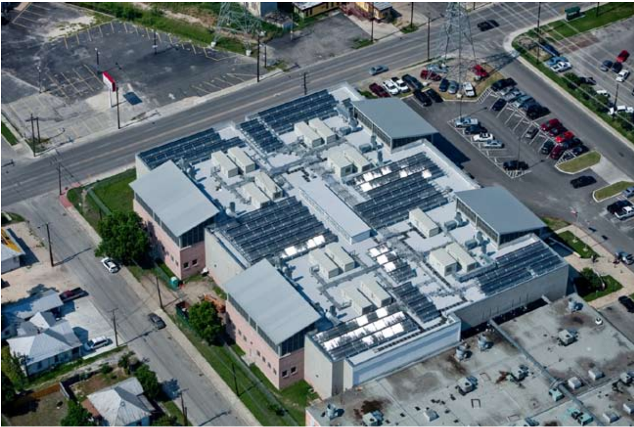
Figure 1 Evacuated tube array on the roof of a jail
